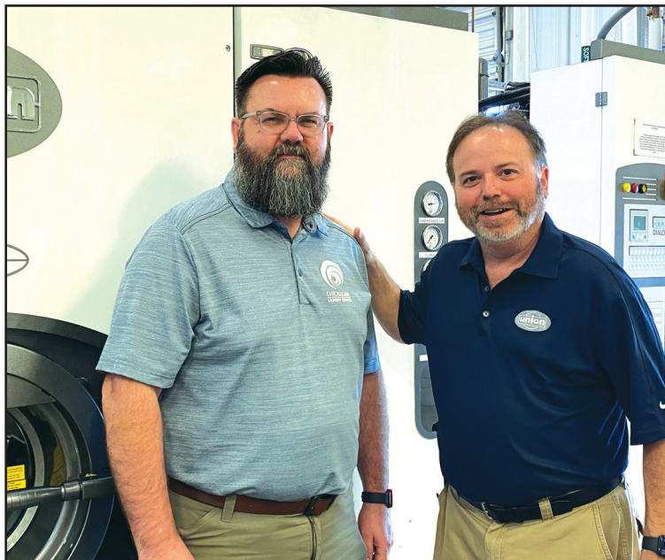
CHICKASAW LAUNDRY SERVICE in Ardmore, OK, recently purchased two Union HL-860 drycleaning machines with solvent heating. Plant manager Brad Houchin (left) is pictured with Matt Lipman of Union Drycleaning Products during the installation and start-up.
